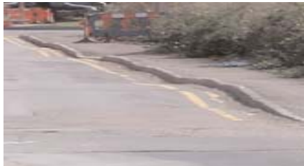
The former land fill site shows obvious signs of settlement (above) and has been leaching contaminants into an adjacent river (below).
