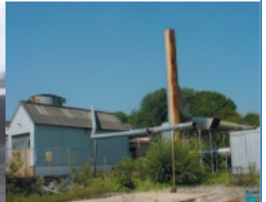
The site had a contamination legacy left by a printing works, a gas works, pigment manufacturing and filled brick pits.
